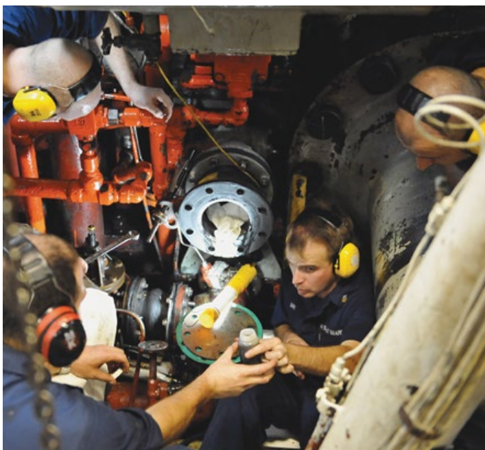
Problem: Taking oil samples in cramped and hazardous conditions without proper cleanliness precautions.
